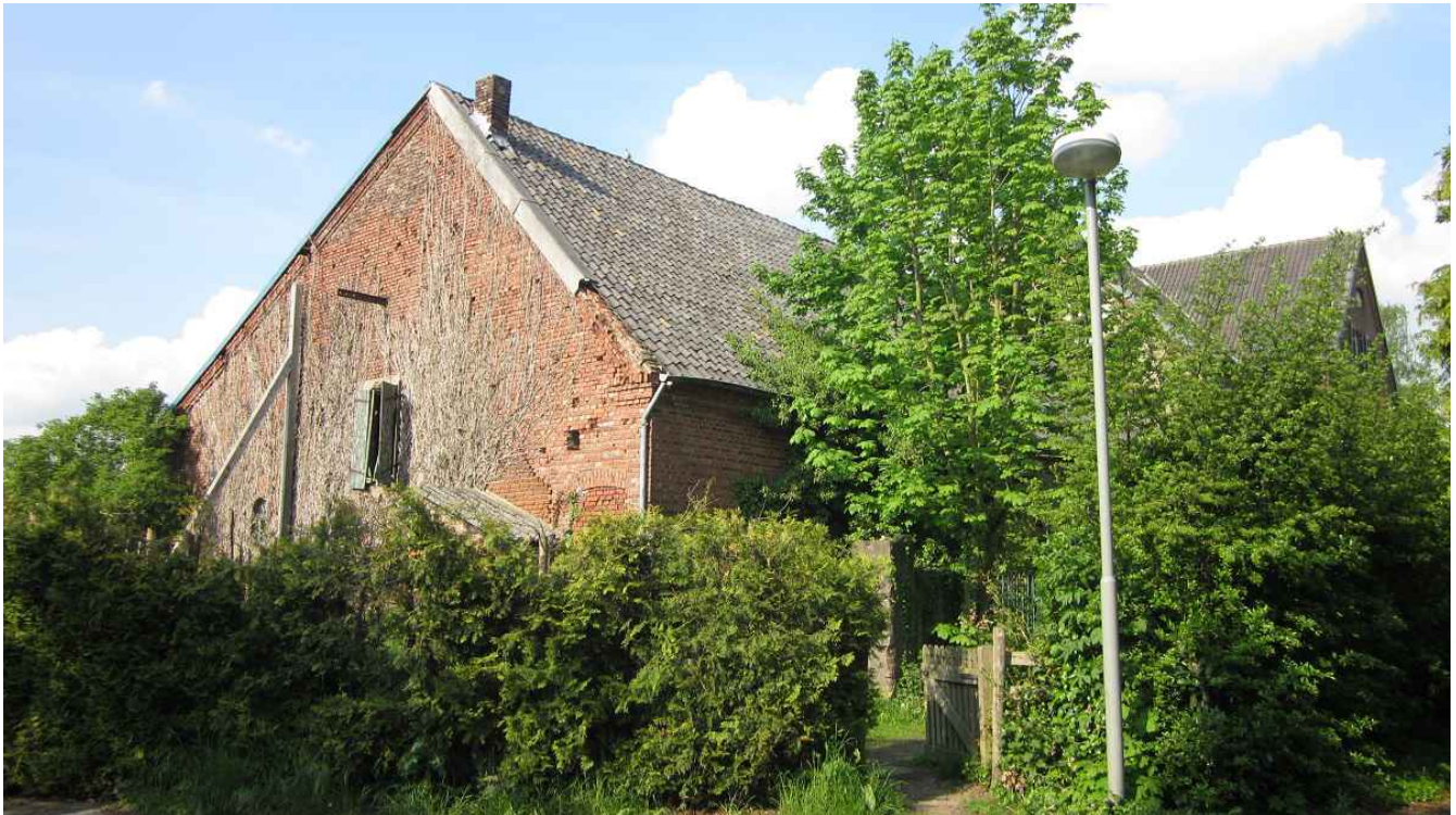
The backside of the Fortress House, the last German stronghold in Bienen. This part of the house faces the dyke over which 'D'Coy, North Novas tried to rush into the village.
