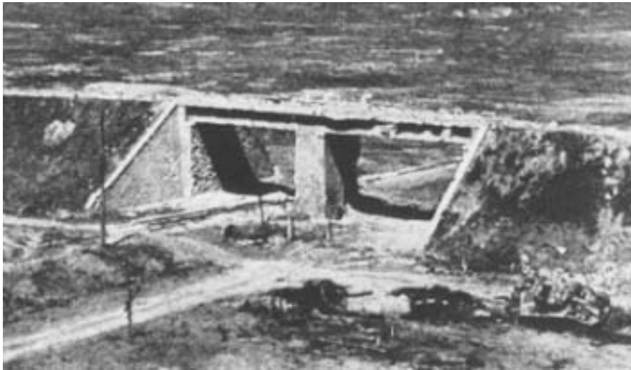
The Flyover (First Overpass)
